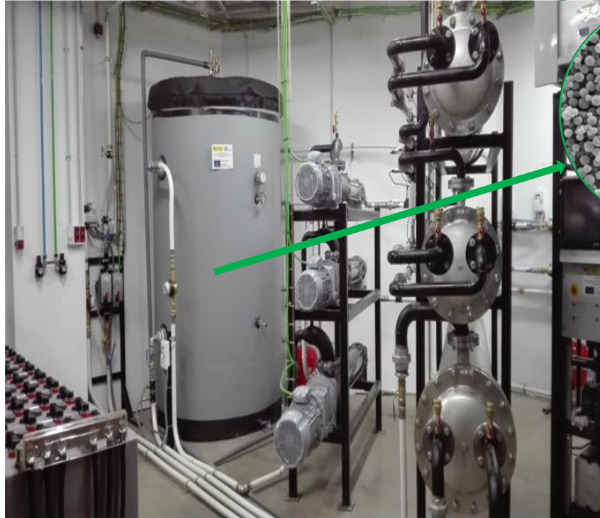
Shell/Tubes Exchanger Water + PCM Slurry Circuit
